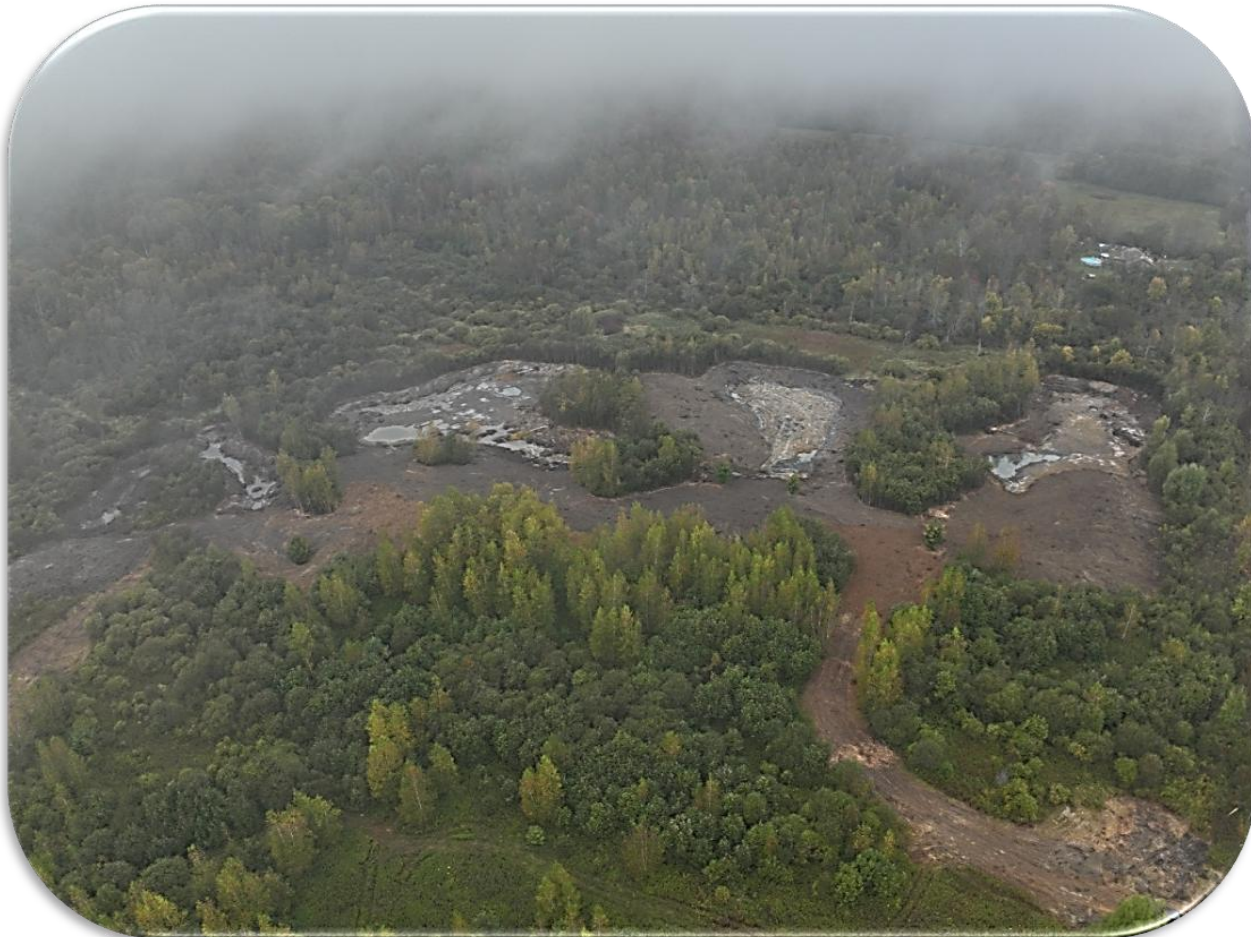
Wetland Construction Site, The Healing Place (SNC 164), September 30, 2026
