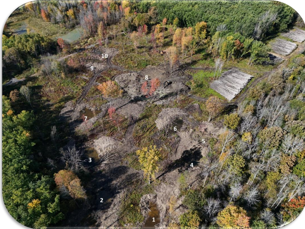
Wetland Construction Site, Two Creeks Forest Conservation Area, October 9, 2026
