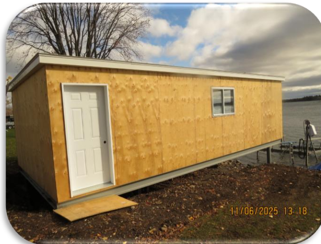
Boathouse on the St. Lawrence River, South Dundas
