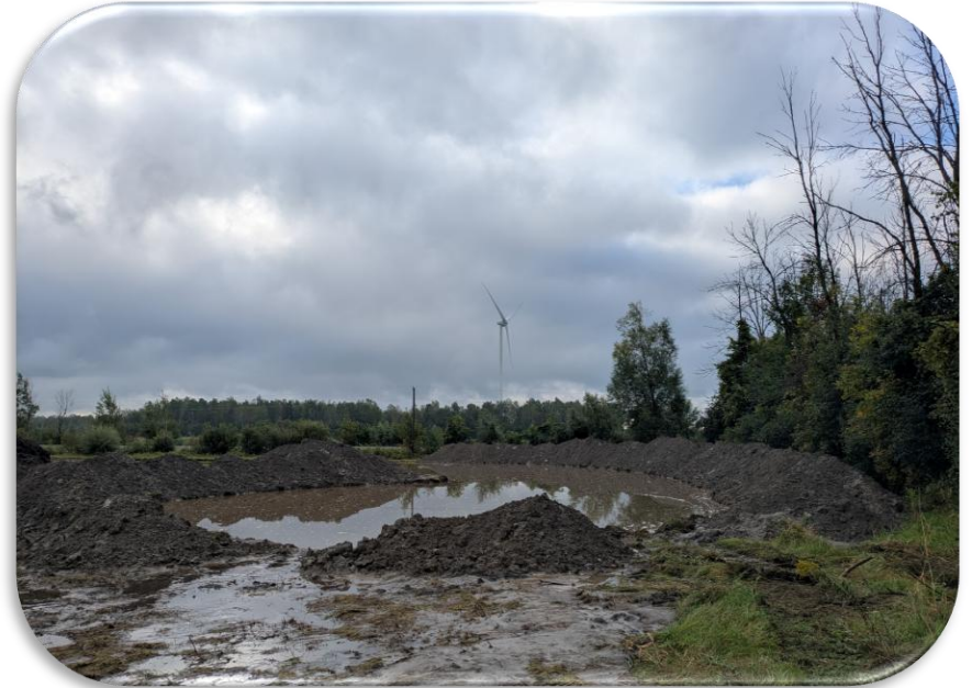
Flooded out – September 3rd, 2026
