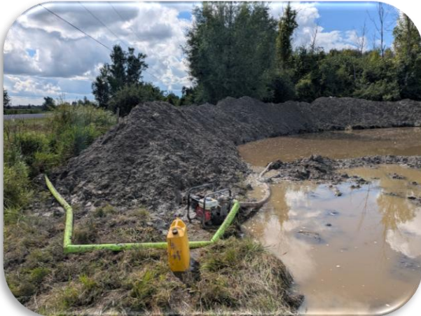
Pumping out the site – September 3rd, 2026
