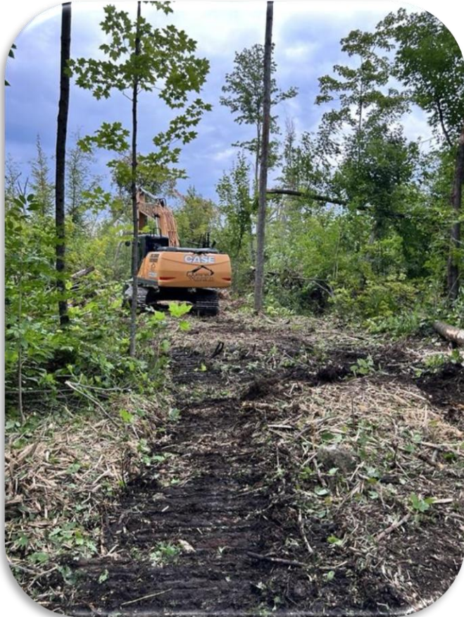
Woodlot Storm Recovery, site preparation Navan, City of Ottawa
