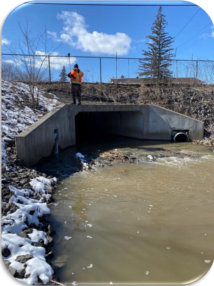
Structure survey in South Castor River
