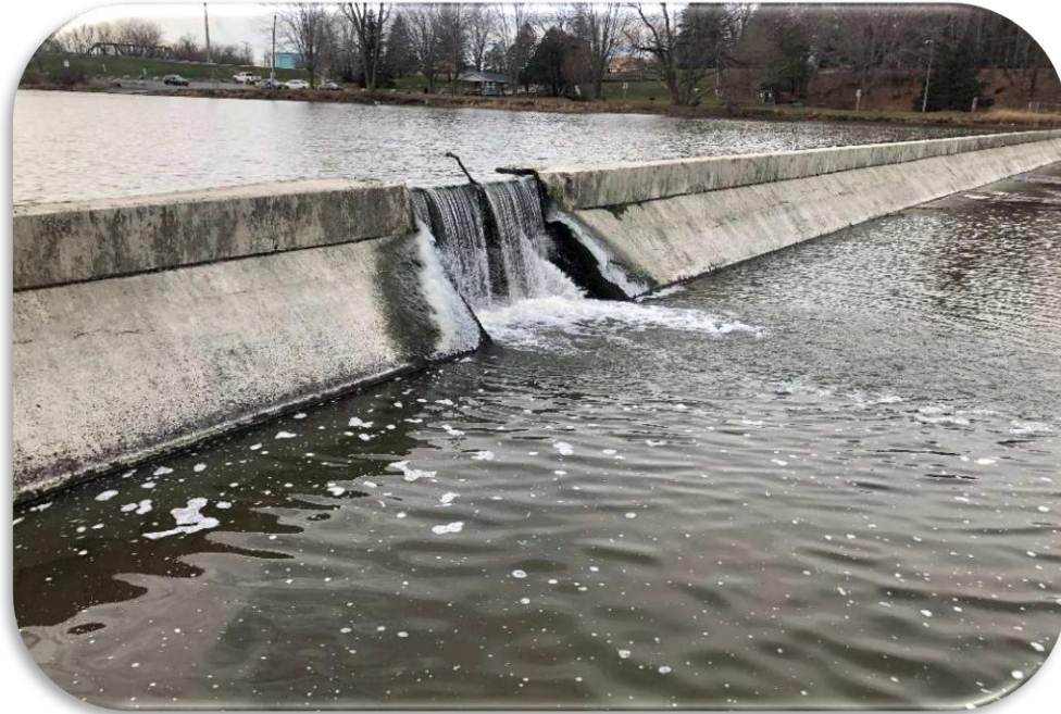
Casselma Weir Sluiceway, winter 2020-2021
