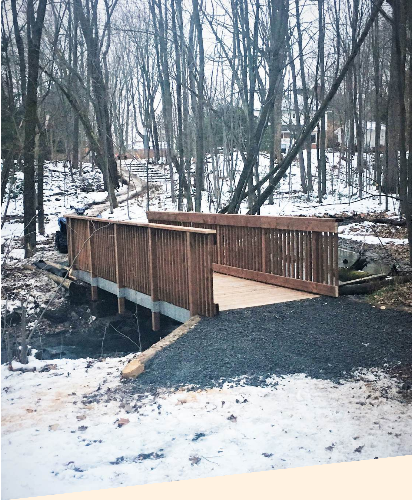
SNC INSTALLED A NEW FOOT-BRIDGE AT J. HENRY TWEED CONSERVATION AREA
