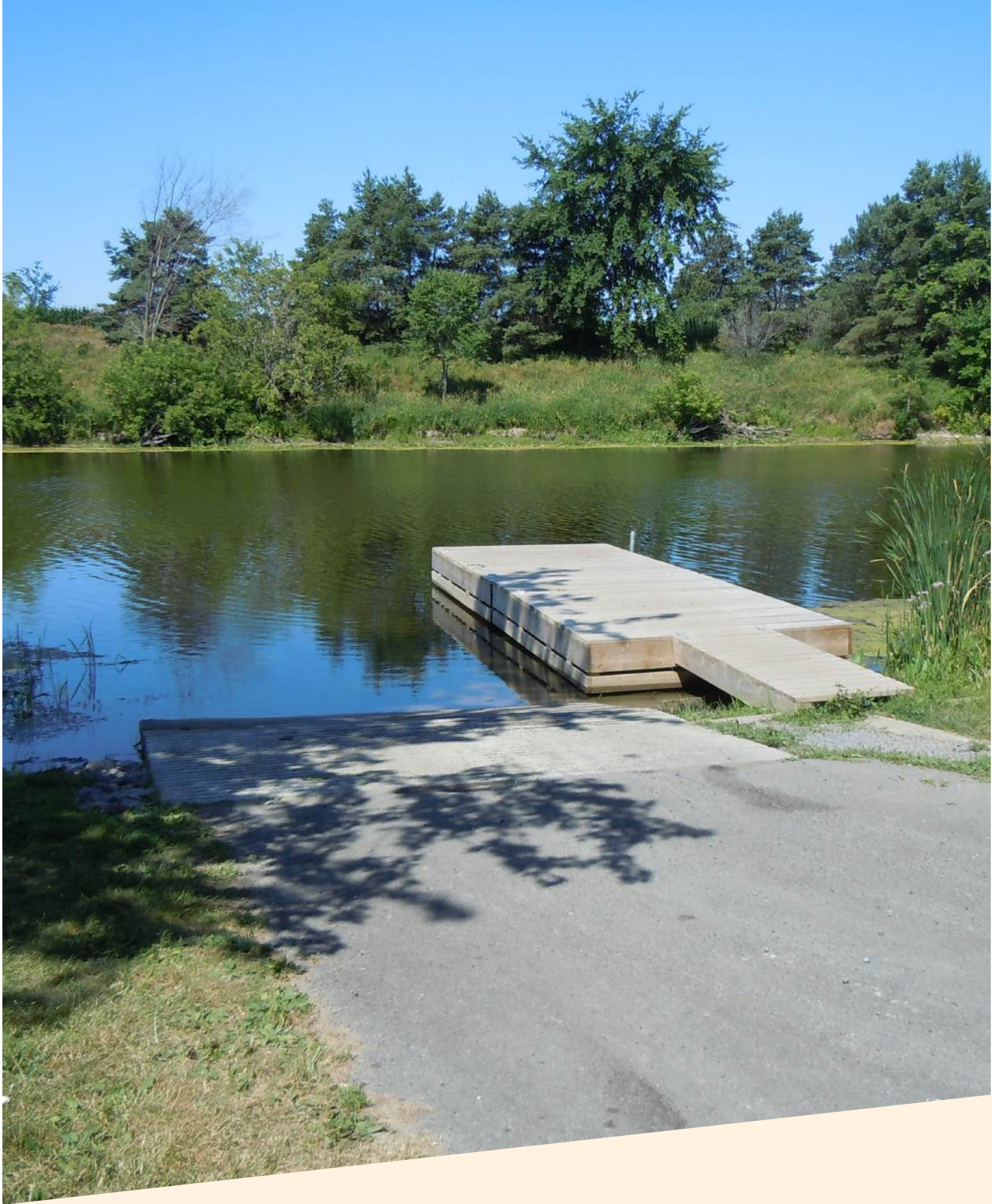
ST. ALBERT CONSERVATION AREA
