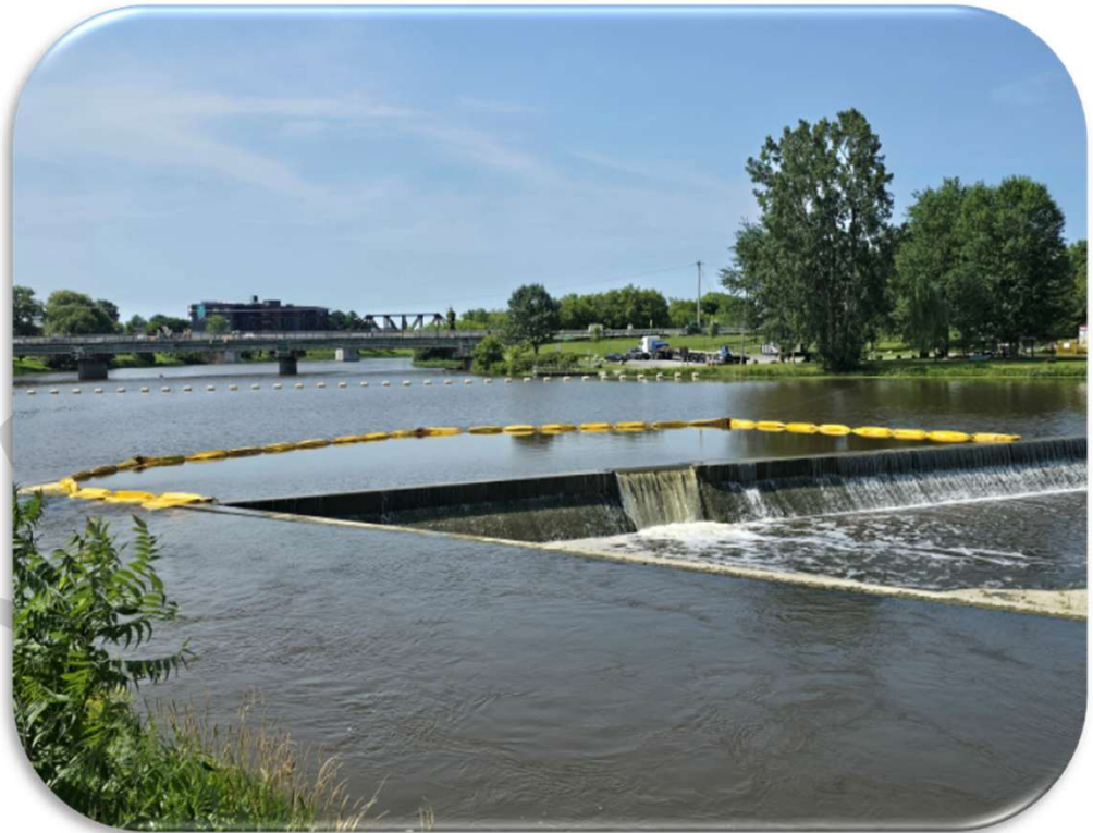
Casselman Dam, July 2026 Casselman
