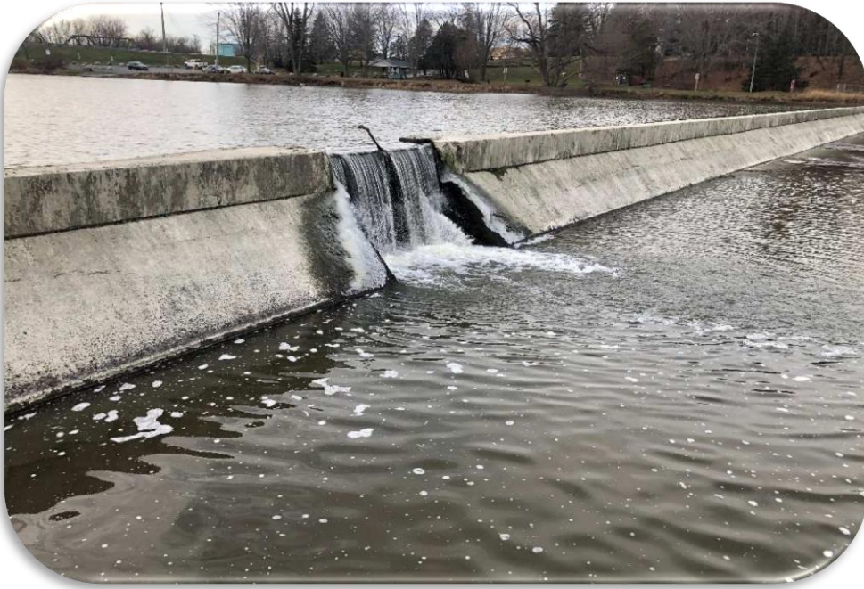
Casselman Weir Sluiceway, winter 2020-2021
