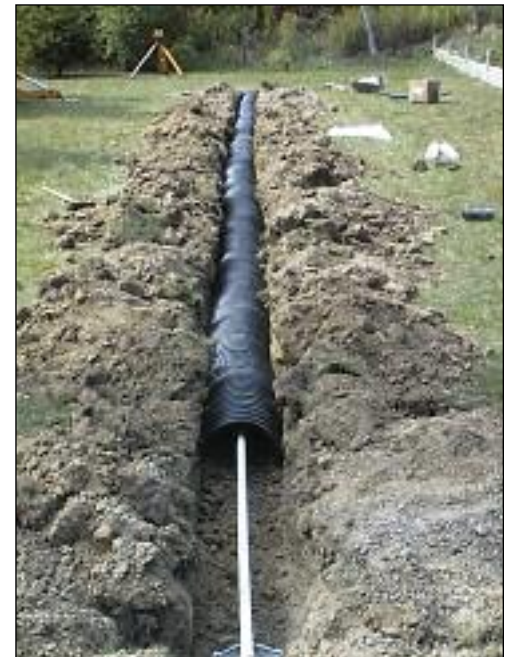
Single line shallow buried trench.
