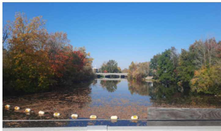
Chesterville Dam, Township of North Dundas
