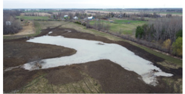
Completed excavated wetland pond on private property, Municipality of South Dundas
