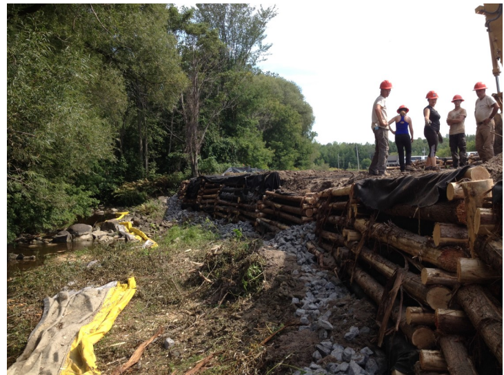
Newly constructed crib wall
