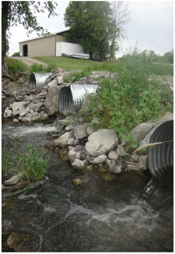
A triple-perched culvert was identified along the stream that could be improved to allow more effective fish migration in low water flow times.
