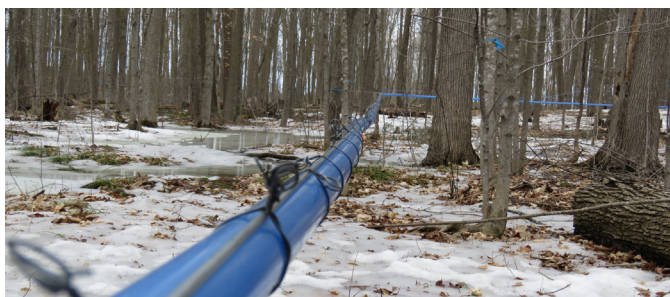
Pipeline through Oschmann Forest in North Dundas
