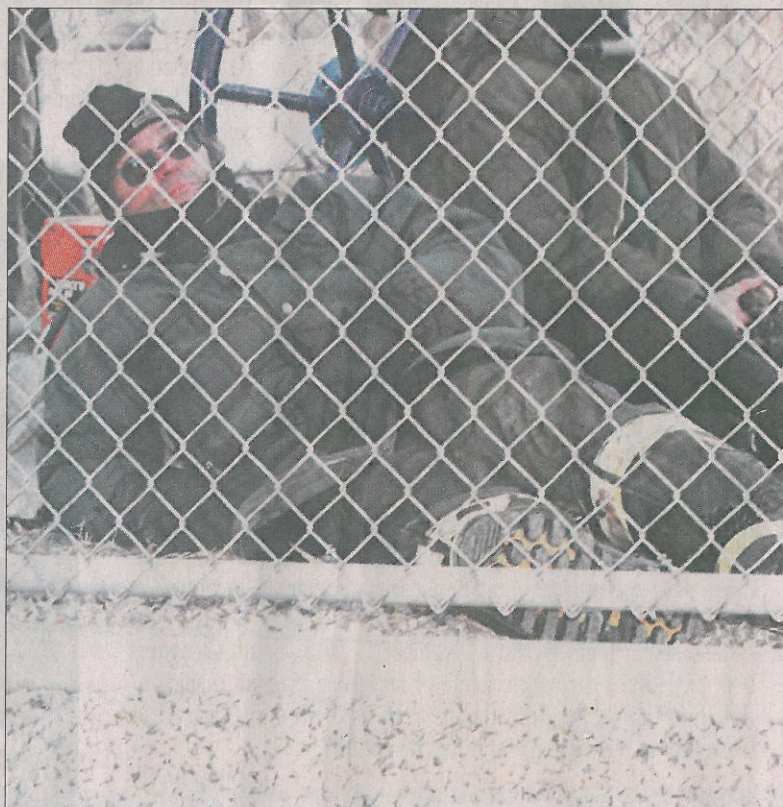
Three protesters chained themselves to an Enbridge natural gas pipeline near Dal Mills Monday. Two men had locked their necks to a valve, part of a contentious Enbridge will use to move oil through the district to Montréal. A third had chained self to a fence around the valve station. The demonstration, which began at ended Monday afternoon when Sûreté du Québec officers removed the protester the site. The Line 9 plan has drawn opposition from people who are worried about project's potential impact on the environment. More inside STEVEN WARRINGTON
