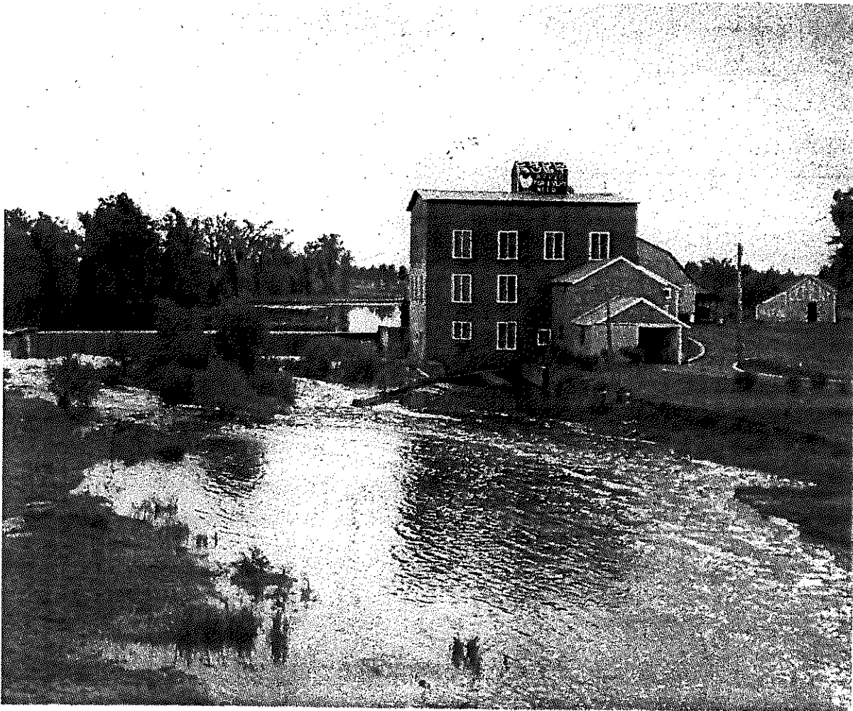
Dam and mill on the South Nation, at Spencerville.
