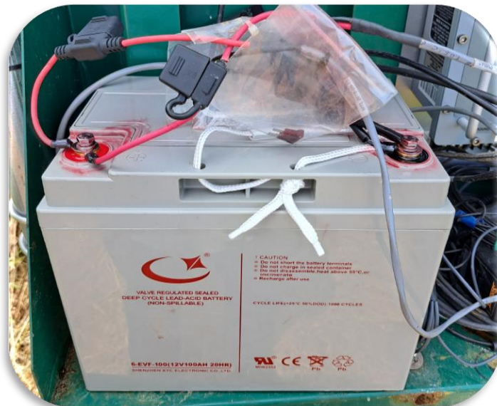
Newly installed replacement battery
