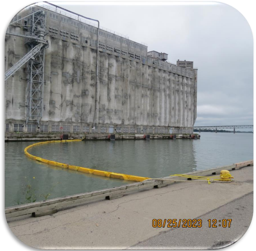
Large Turbidity Curtain deployed with flotation devices and anchored to land on both ends
