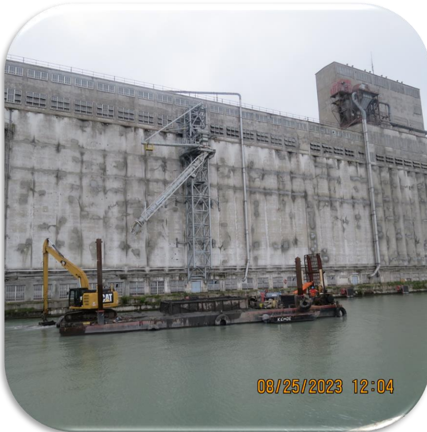
Dredging was conducted via an excavator mounted on top of a barge.
