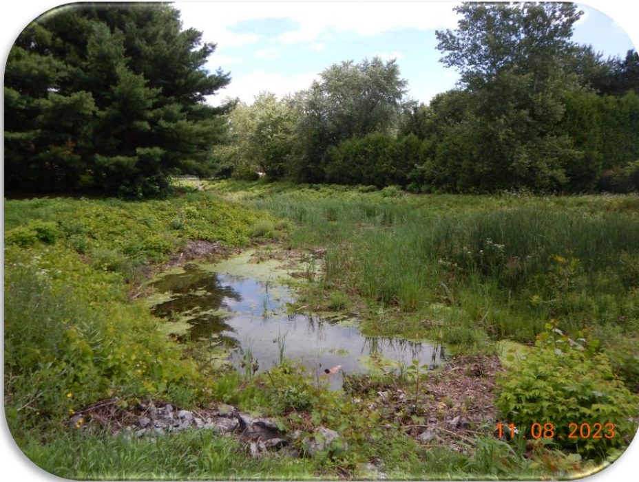
Olde Town Road stormwater facility, Russell.
