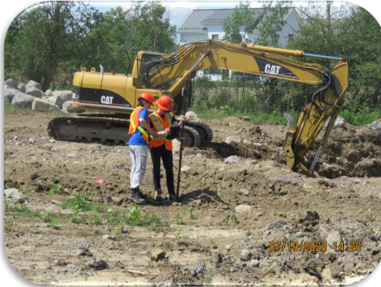
Construction inspections, Metcalfe, City of Ottawa
