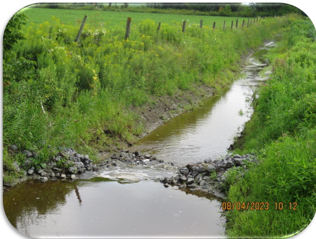
Staff working to looking into erosion concerns near Plantagenet
