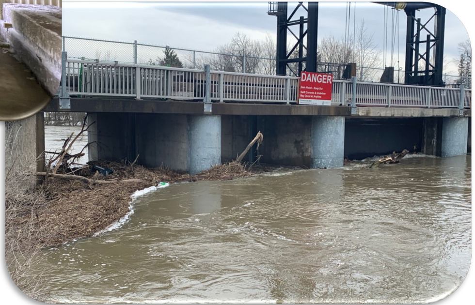
Debris at dam due to ice storm and tree damage
