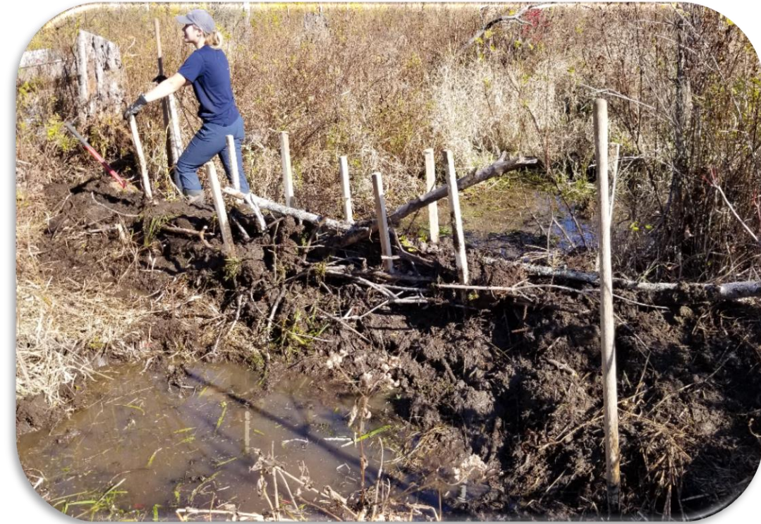
Beaver Dam Analog (BDA) constructed on private property near North Plantagenet, Oct 24
