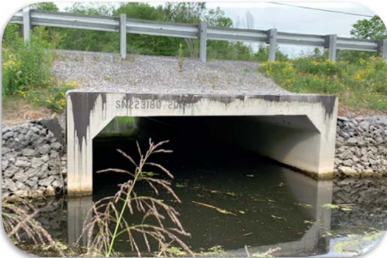
Concrete box culvert located on South BB tributary
