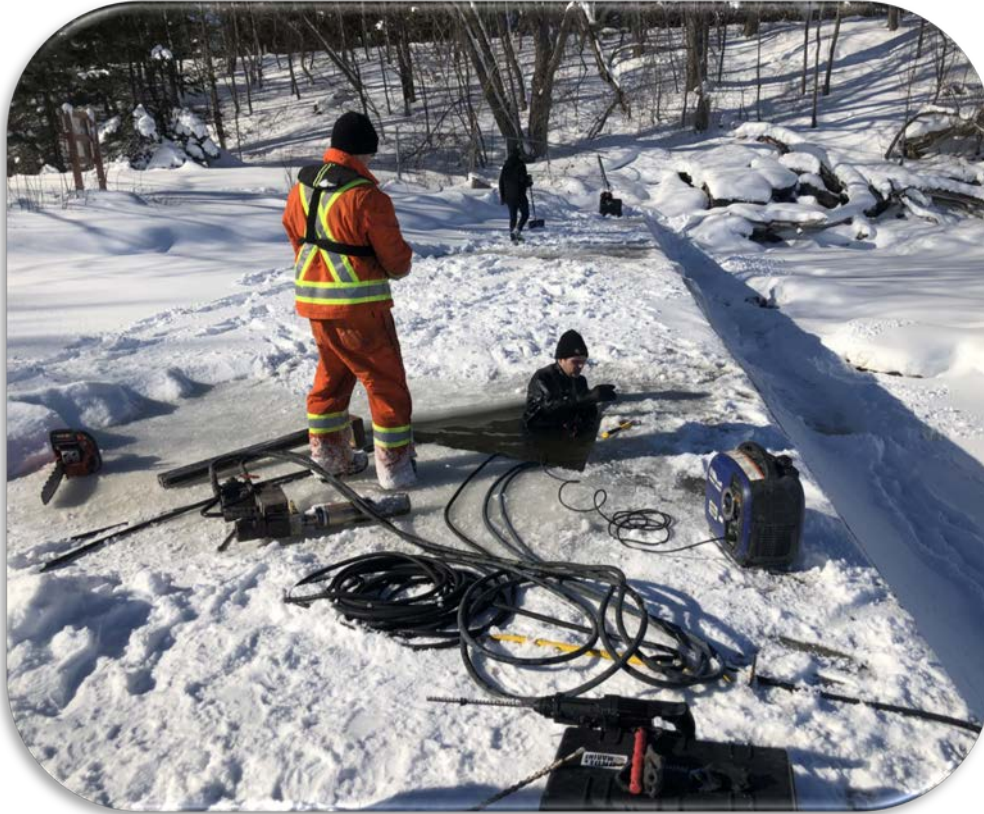
Divers taking core samples from the Casselman Weir
