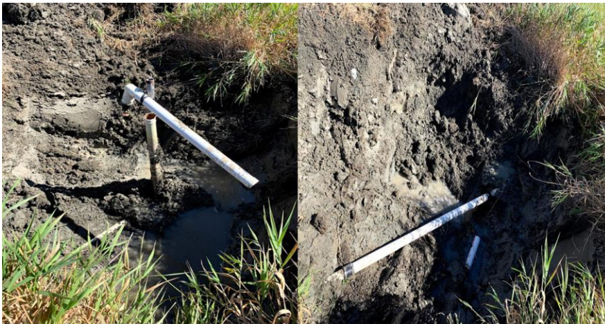
Picture Caption: Repaired dosing line from Alfred lagoon to wetland header pipe.
