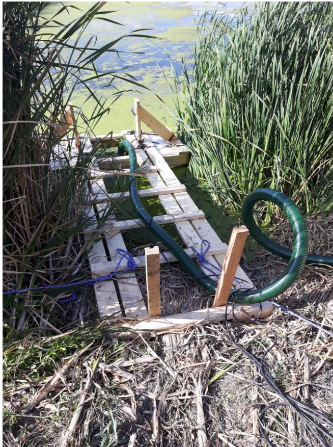
Picture Caption: Floating dock with \frac{3}{4} HP sewage pump installed in Alfred municipal lagoon
