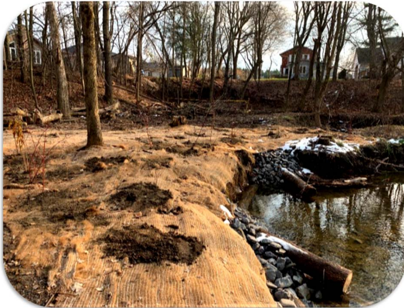
J. Henry Tweed Conservation Area 2019 shoreline restoration project
