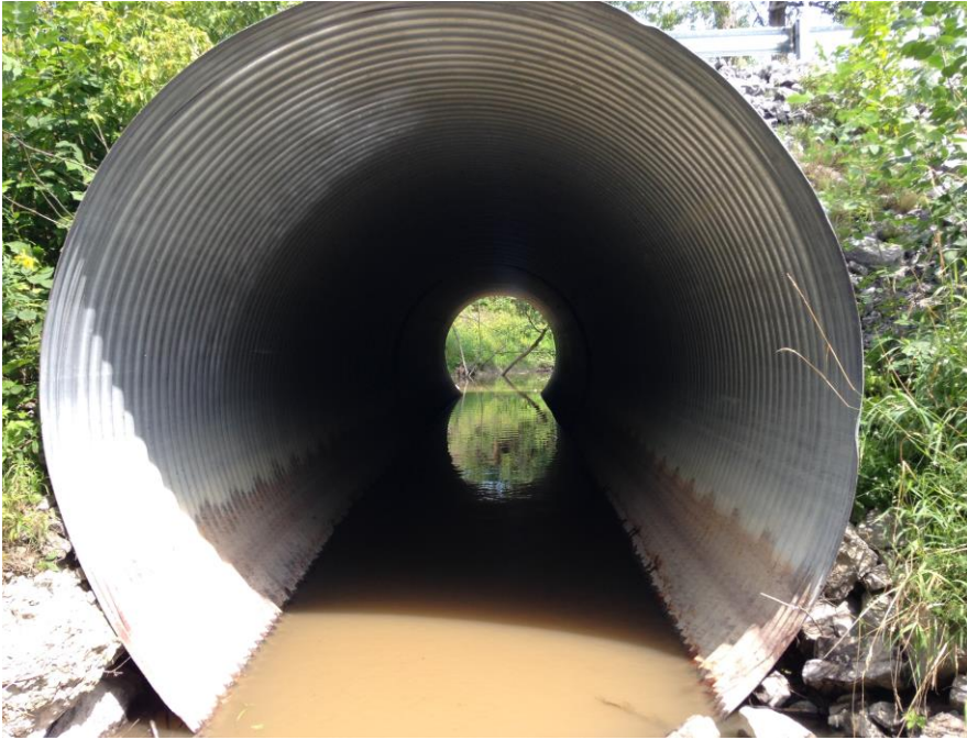
Culvert 35 – 119 Interior view
