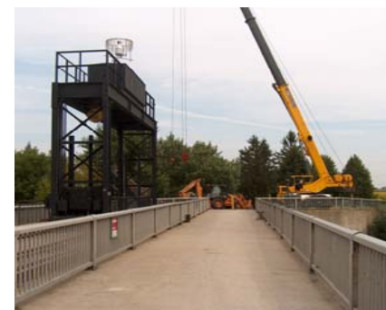
Repairs to the Chesterville Dam
