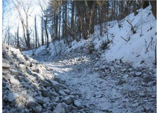
The Bourget Municipal Drain, located on County Road 8, has steep banks which have eroded over time creating hazardous conditions for the house located approximately 20 meters from the top of the bank. Kollaard Associates was hired to prepare a geotechnical report detailing the methodology of the bank restoration. Since SNC partnered with the UCPR for this project, the UCPR Public Works department executed the proposed methodology.
