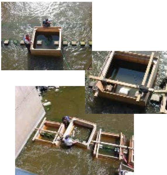
**Placement of Blasted Rock:** Undertaken by SNC in 2005, this project consisted of the placement of riprap in a large hole (16m x 10m x 1.5 m (depth)) immediately downstream of the Chesterville Dam's concrete apron area. The material used was riprap free of fines with average nominal sizes of 18" to 24", with no more than 25% greater than 24". The riprap was placed using a crane, until the grade of the riprap was the same elevation as the grade of the concrete slab.
