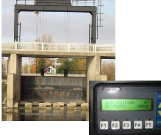
**Loglifter Repairs:** The loglifter is used to haul the logs up and down in the 4 bays at the Chesterville Dam. In 2005, the arm of the loglifter was repaired.
