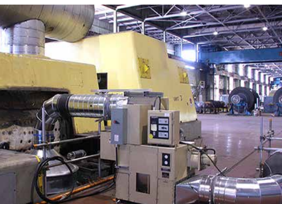
A dehumidified air system at Lambton GS minimizes corrosion of the turbine shaft and blades.
