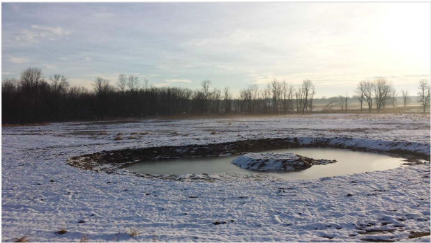
Pond completion— December 2016 Transporting the material off site was the most significant project cost, the innovative contractor created “islands” to deposit clay increasing habitat diversity
