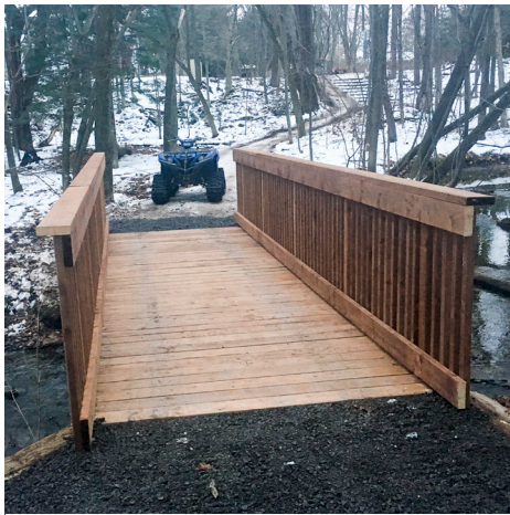
New bridge at J. Henry Tweed CA
