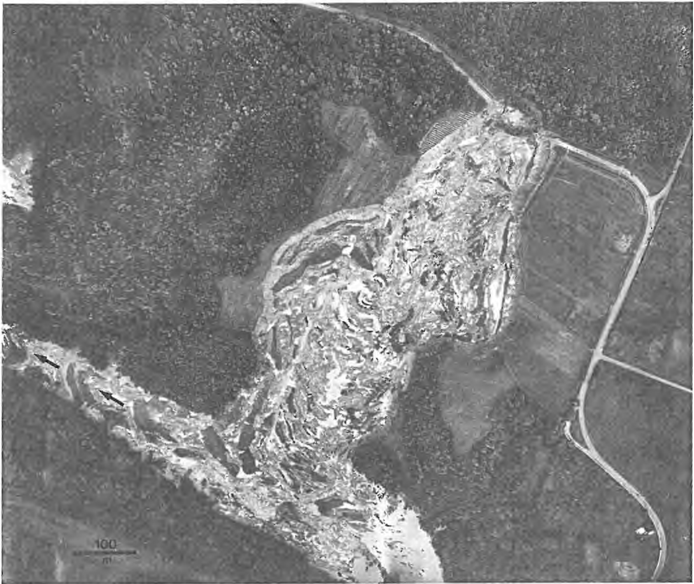
Fig. 5. Vertical aerial photograph of the 1993 Lemieux landslide taken on June 22, 1993 (courtesy of South Nation River Conservation Authority). Direction of flow of South Nation River is shown by arrows. Scale is approximate.
