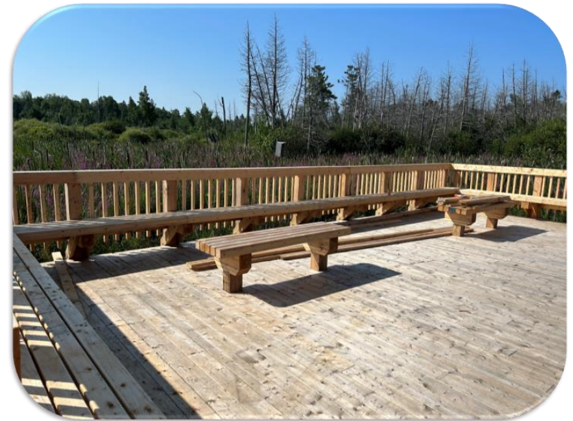
Findlay Creek Boardwalk Extension City of Ottawa
