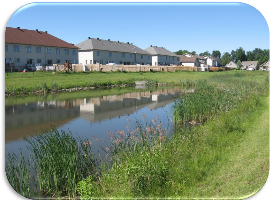
Stormwater Facility The Nation Municipality
