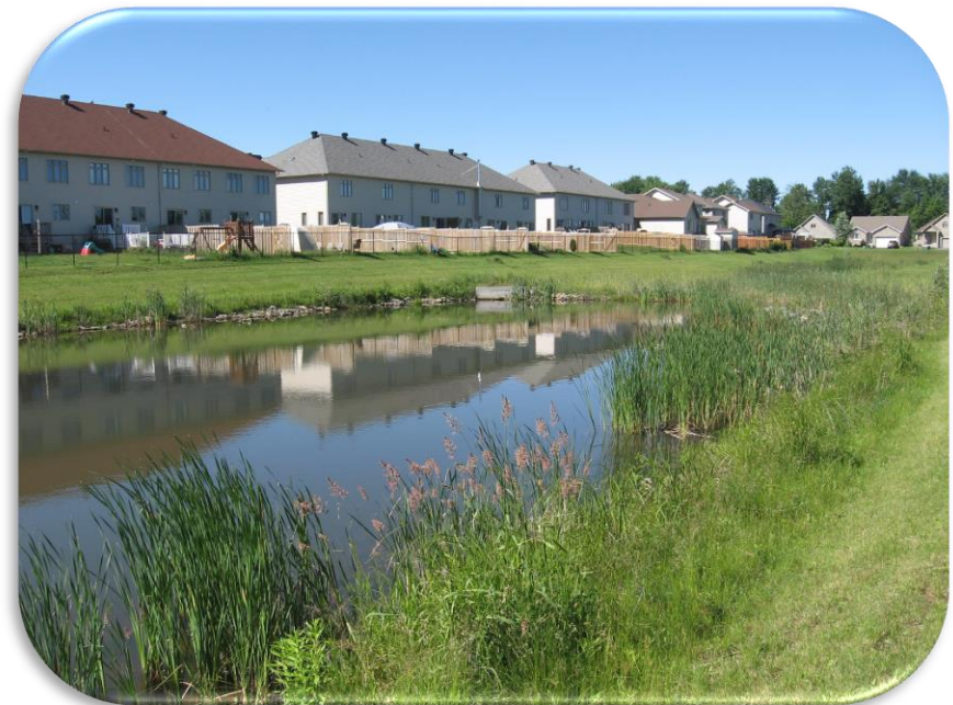
Stormwater Facility The Nation Municipality
