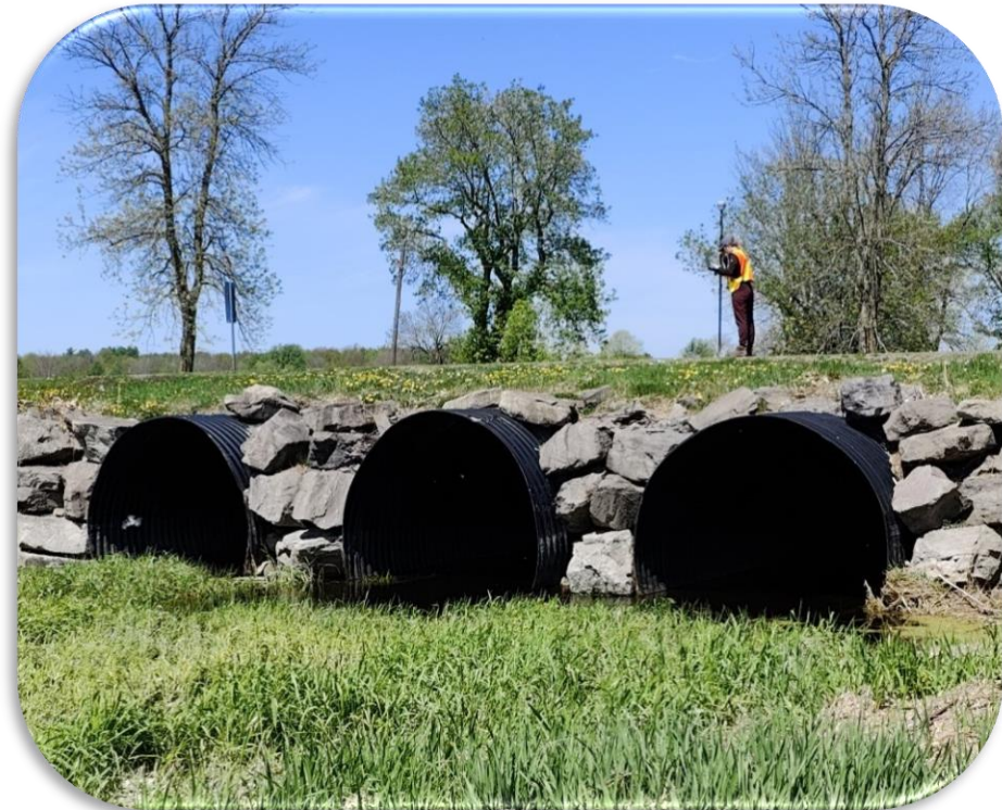
Public infrastructure survey Township of South Dundas
