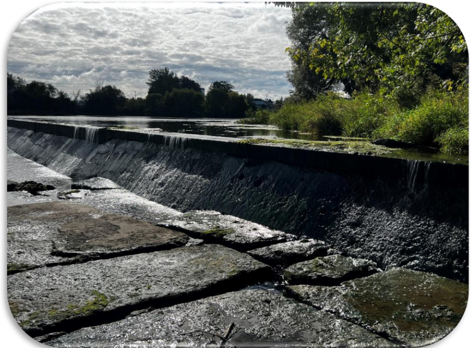
Casselman Dam Nation Municipality
