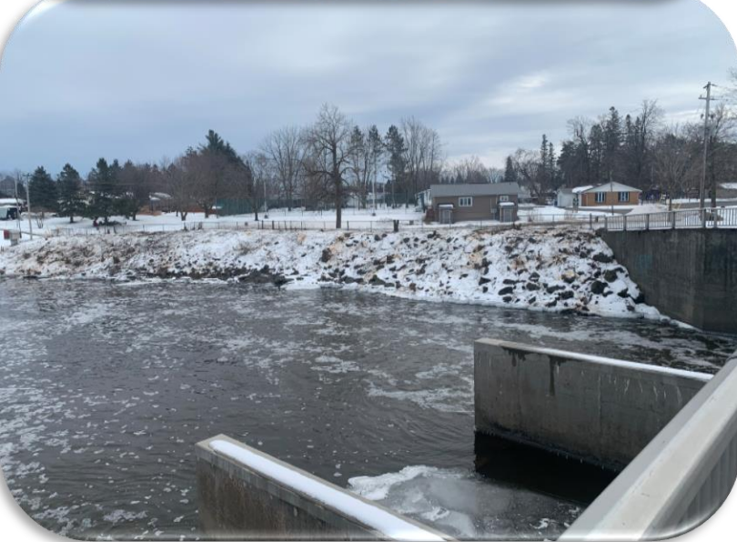
After tree removal
