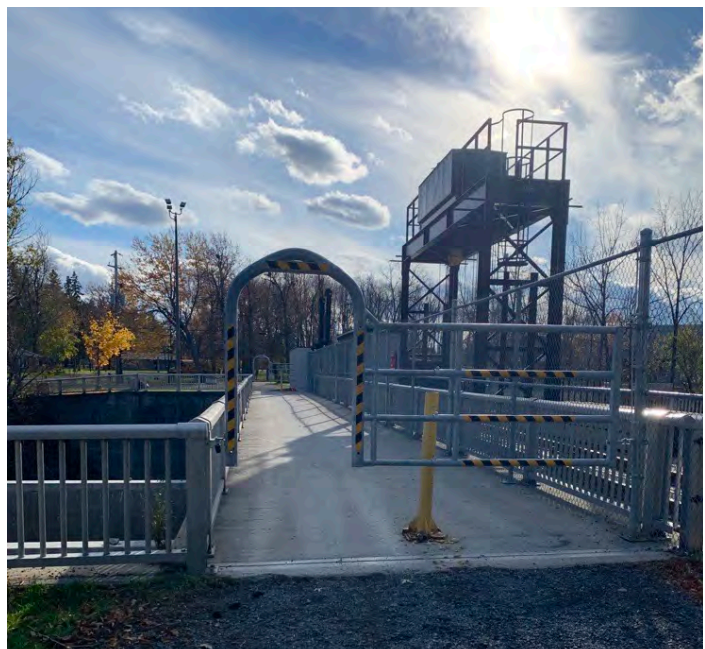
New Pedestrian Walkway Gates, Chesterville Dam, Township of North Dundas
