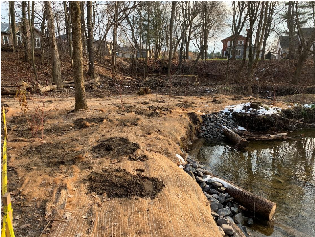
Figure 9: Coconut Matting and Plant Material Installed at Second Erosion Site
