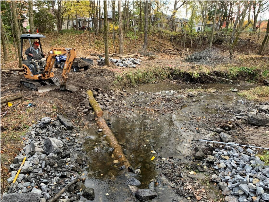
Figure 8: Log Vane Installation at Second Erosion Site
