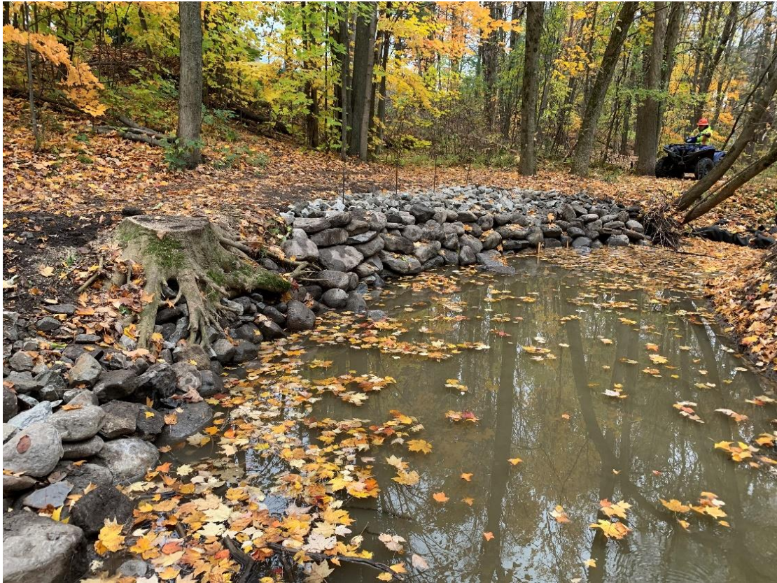
Figure 7: Completed Shoreline Stabilization at First Erosion Site
