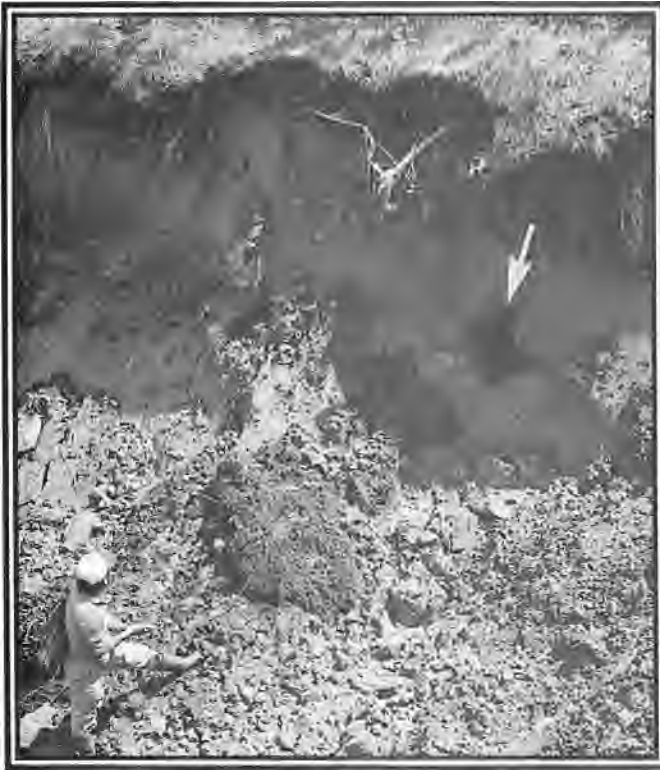
Figure 8. Indicative of the high water table at the time of the landslide, there was widespread standing water and evidence of drainage into the subsoil on the undisturbed surface around the margin of the crater. After the failure, groundwater seeped from the crater sides, with horizontal pipes being eroded at locations of concentrated flow. Pipe diameter ranged from 0.1-1 m and most were located at a depth of about 2.5 m at the sand/ silt interface. The pipe in this photograph was located at the headwall of the crater where eighteen active pipes were observed on Thursday, June 24, 1993. Many of these pipes continued to enlarge in diameter and depth over the summer. GSC 1993-295B
